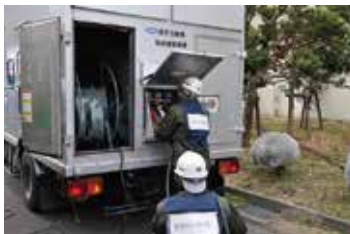
Power supply vehicle connection drills
